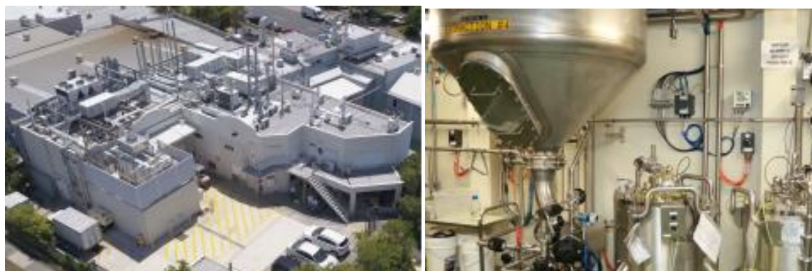
Figure 5 – Southport manufacturing facility up and running
